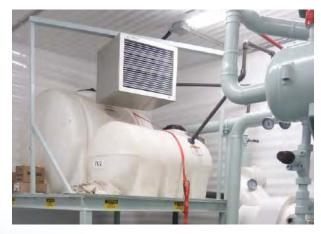
• A 10 KW electric industrial heater maintains a minimum 55° F (13° C) room temperature.
