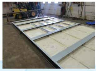
• The bottom of the structural steel base is insulated with 3" spray foam insulation.
